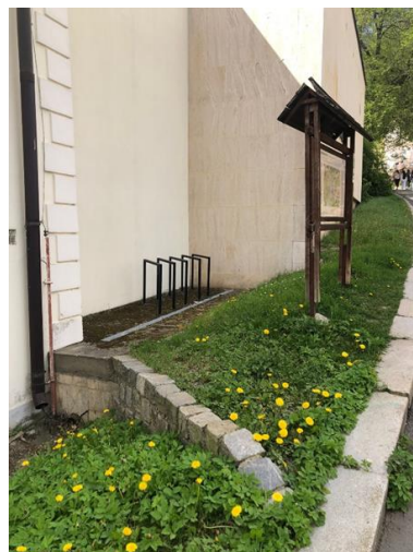
Figure 5: Bad examples of cyclist infrastructure. The bike stands are not usable (too close to the wall and not accessible). The path on the right, although clearly separated from cars and pedestrians is too narrow, endangering pedestrians on the side walk.
